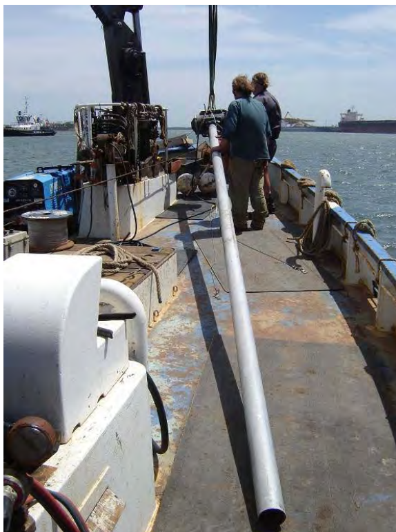
Photo 2. Vibrocoring from the crane barge "Alkira".
