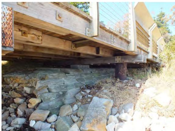
**Figure 7.13** Archaeological remains of a sandstone wharf pier or abutment are protected by a new timber deck.
