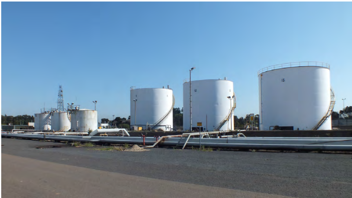
Figure 6.30 Three tanks (left) on the north side of Road L, installed in the 1950s, may become redundant. Three tanks (right), also installed in the 1950s and early 1960s, would remain in use with no works required.
