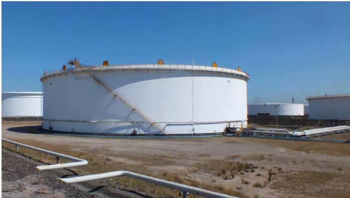
Figure 6.28 View of a cone roof tank in the Western Tank Area, installed in the 1970s.
