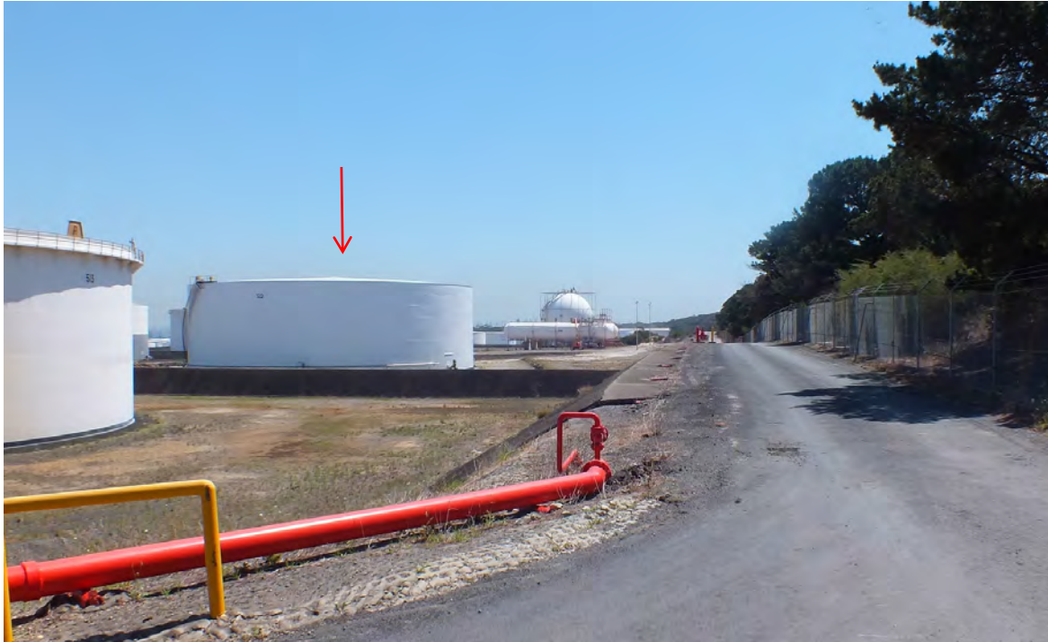
Figure 6.18 View along the eastern boundary of the Site, towards the north. The large cone roof tank indicated (red arrow) would be converted from intermediate product storage to finished product storage.
