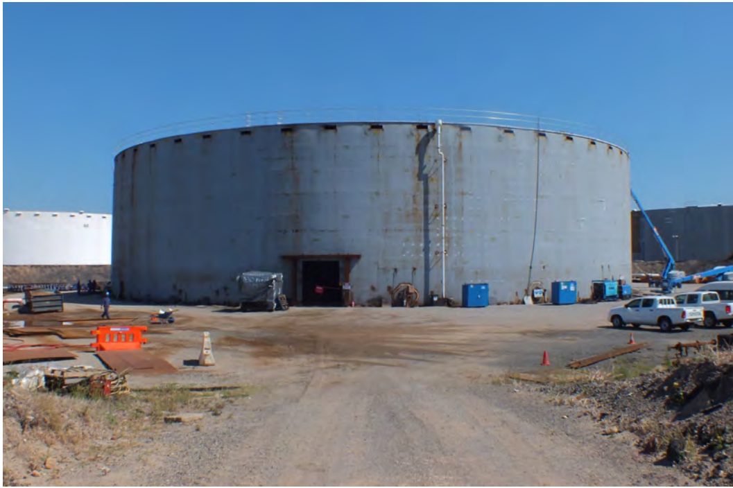
Figure 6.15 A tank in the Western Tank Area undergoing conversion. Insulation panels have been removed and the tank floor is being rebuilt.
