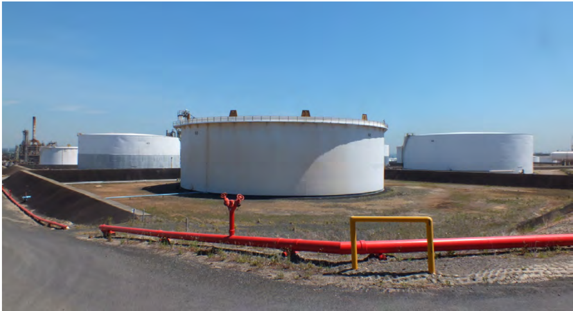
Figure 6.13 Tanks in the Eastern Tank Area, installed in the 1950s to 1970s. The photo includes examples of tanks with fixed cone roofs (right) and floating roofs (centre).
