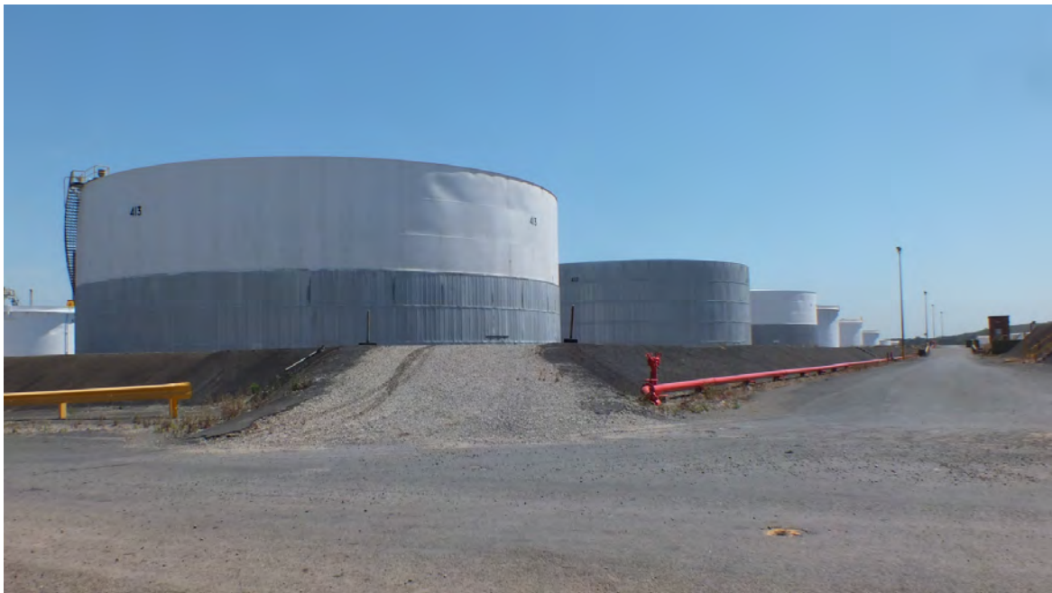
Figure 6.19 View of tanks along the west side of Road 2. Three tanks are partially or fully insulated; this insulation and associated steam and condensate nozzles would likely be removed.
