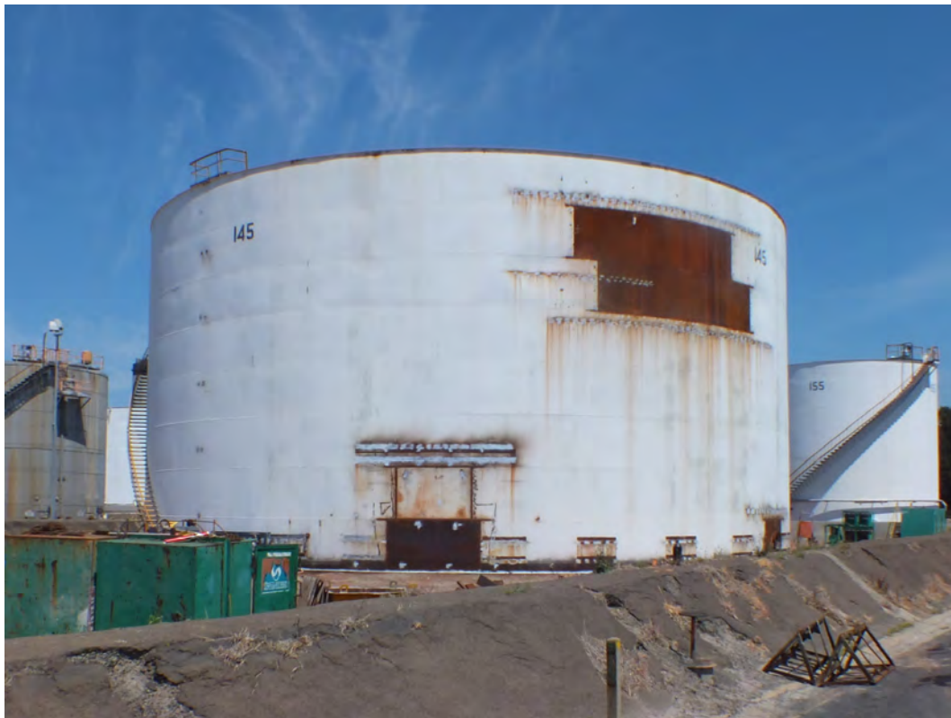
Figure 6.14 A tank in the Eastern Tank Area undergoing maintenance, including replacement panels.
