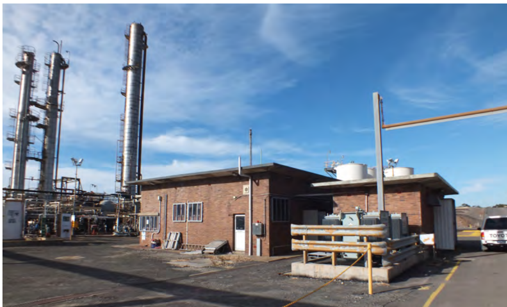
Figure 3.19 Plant 36 Control Room and associated Motor Control Centre, 2012. This building was constructed in c1961 in association with the Alkylation Plant. All but one early control room on the Site would be demolished.
