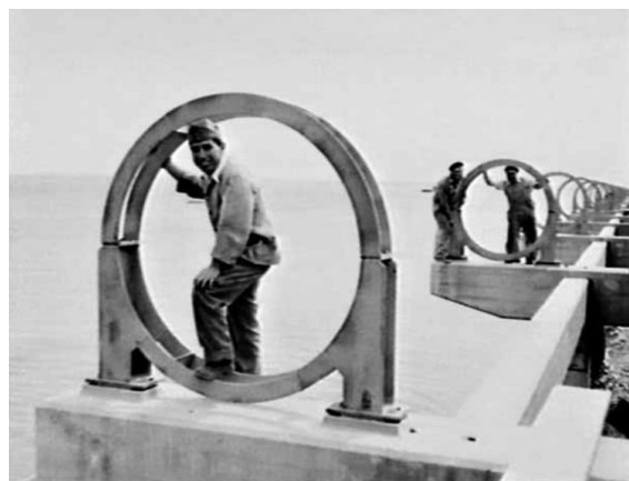
Figure 3.14 AOR wharf pipeline construction, showing steel pipe brackets, 1954; photo by Jack Hickson (Source: NSW State Library, Australian Photographic Agency – 42955).
