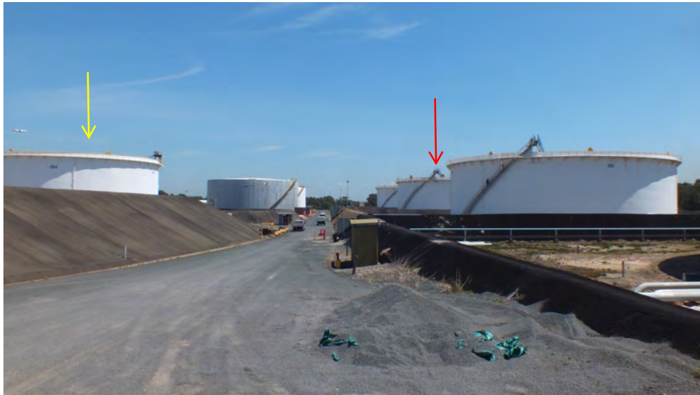
Figure 3.6 View of four large floating roof tanks along the northern boundary of the Site (right), in the Eastern Tank Area, 2012. Three of these tanks were constructed in approximately 1955 and are original to the Site; the tank indicated with a red arrow has since been replaced with a similar tank in the same location. These tanks would be retained. One large floating roof tank on the south side of Road B (left, yellow arrow), constructed between 1955 and 1961, would also be retained.
