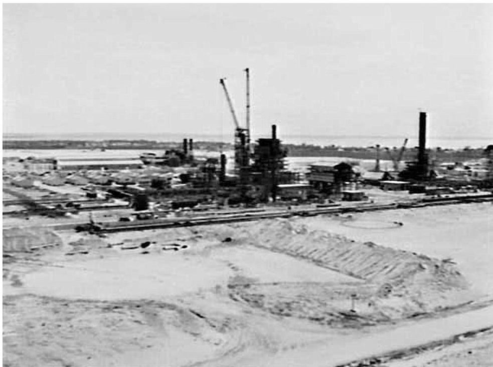
Figure 6 Australian Oil Refinery under construction, 1954 (Source: State Library of NSW, Australian Photographic Agency – 42956).
