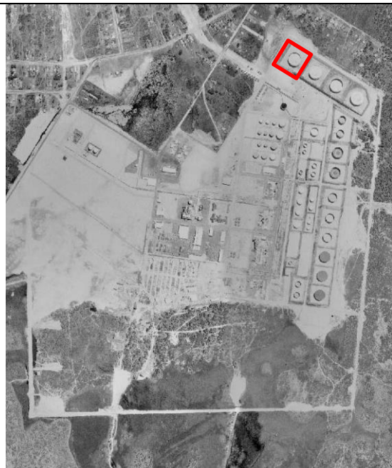
Figure 7 Australian Oil Refinery during construction, 1955 (Tank 101 outlined in red) (Source: Sutherland Shire Maps).
