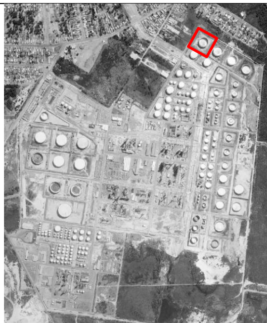
Figure 10 Australian Oil Refinery 1978 (Tank 101 outlined in red) (Source: Sutherland Shire Maps).
