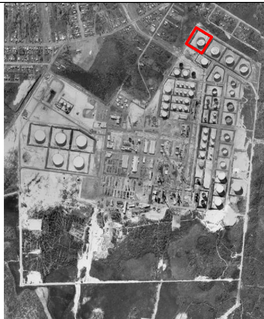
Figure 8 Australian Oil Refinery, 1961 (Tank 101 outlined in red) (Source: Sutherland Shire Maps).
