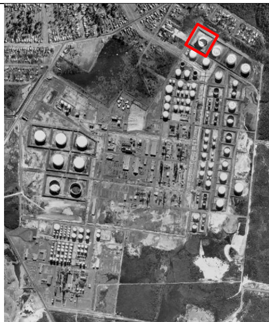
Figure 9 Australian Oil Refinery 1970 (Tank 101 outlined in red) (Source: Sutherland Shire Maps).
